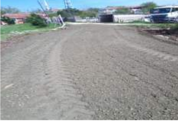
Kavacık Mahallesi 141/2 Stabilize 90 m 2
